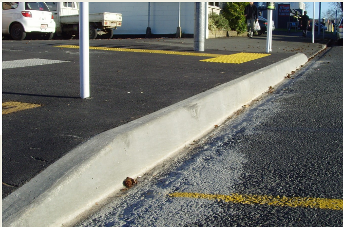
Figure 5: Liverpool Street Stop showing kerb height
